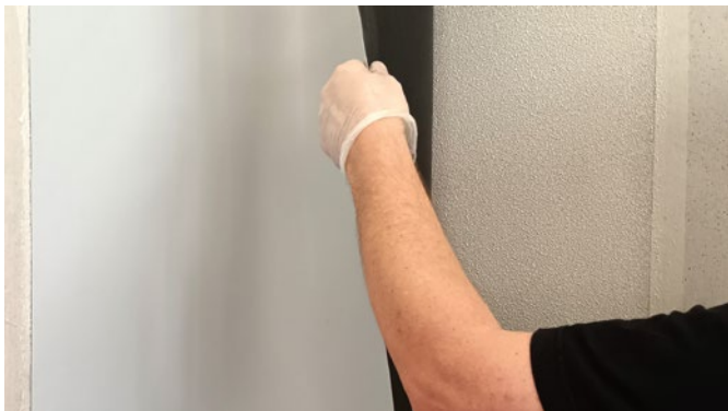
Bonding MODUL covering to the wall from the corner
